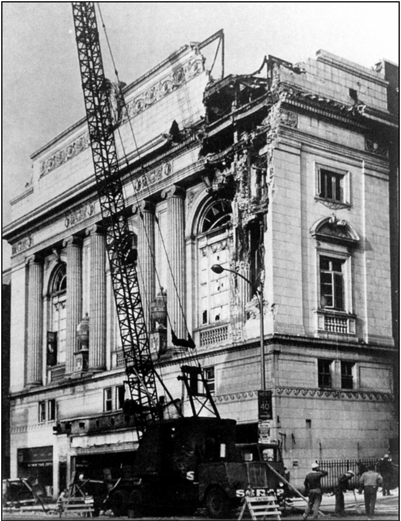
Stanley (later Stanton) Baltimore being demolished 1965
