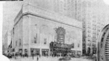
The Stanley, Pittsburgh, built by Hoffman-Henon Company for the Stanley-Davis-Clark Corporation. Complete York air cooling and air conditioning equipment installed.
