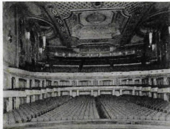
The Fox Theatre, Washington D. C., keeps its house cool and comfortable in hot weather with its YORK air-cooling and air-conditioning equipment. Leading theatres in every section of the country have turned to YORK for the answer to increased summer profits.
